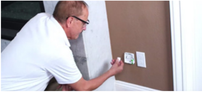
1 Install wall module.
